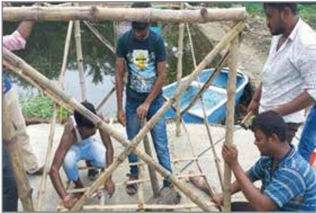
B.F.Sc. Students were involved in Construction and installation of Bamboo Cage in pond
