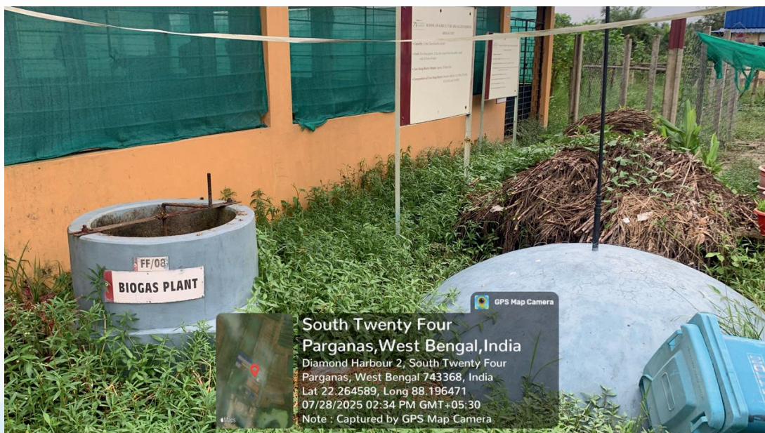
Fig. 2: Biogas Plant utilized for converting organic waste into clean energy and promoting circular resource use
